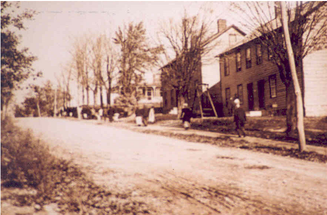
Above: Mill housing along Burden Lake Road
