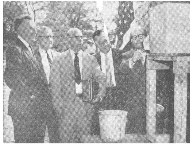
H.H. Butler applies mortar to the cornerstone in 1957 for the high school. Butler donated the land for the school. Others left to right in photo include Carl C. Beck, board member; John DeFreitas, board president; Elmer Stahlman, supervising principal; and Roland H. Trathen, board member.
