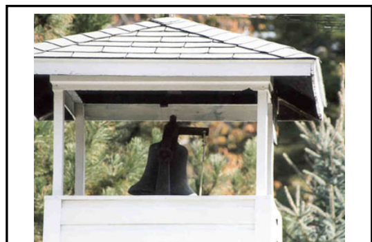
The cupola housing this bell has been restored: details inside!
