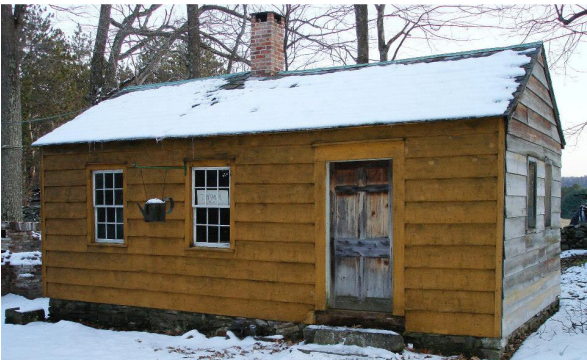
The tin shop as it now stands in Eastfield Village.
